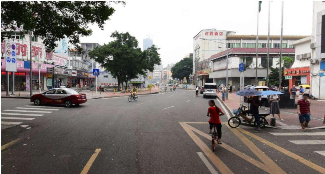
Figure 8. Current condition of Shahe Street- Xinzhong Road.
